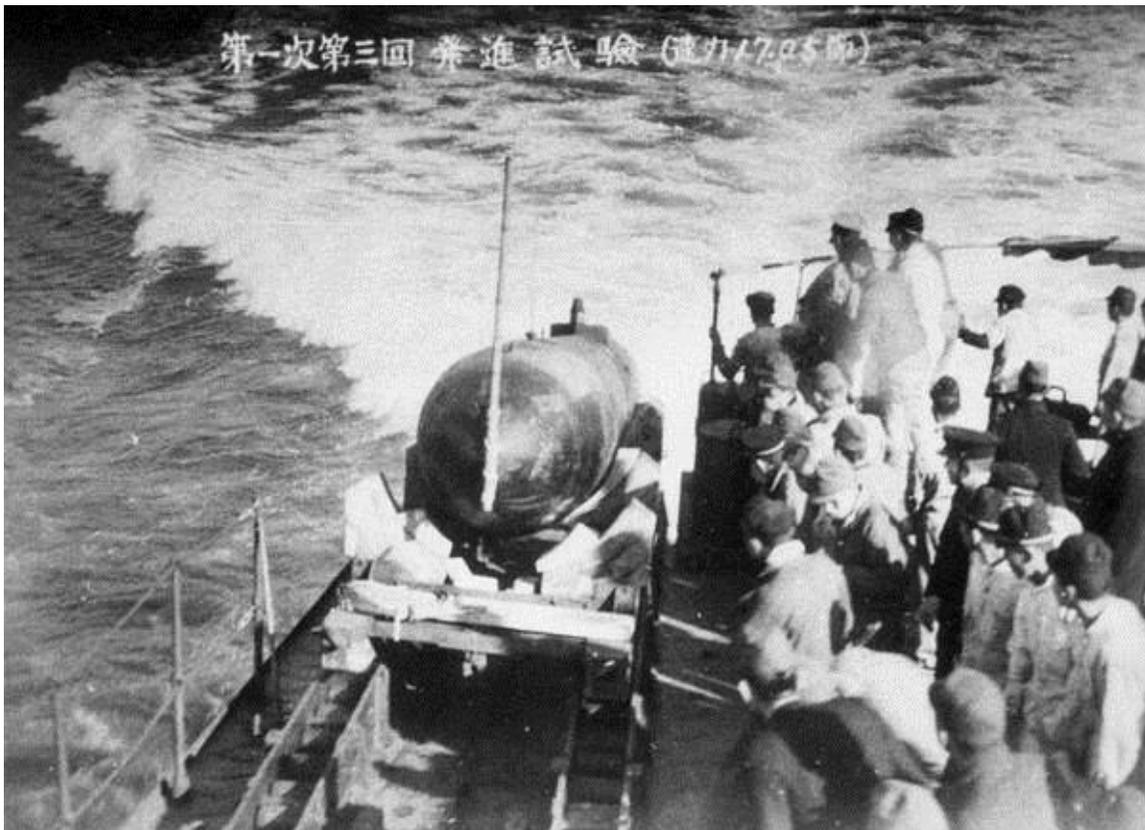
**3.3 Kaiten Human Torpedo:** The Kaiten was a manned torpedo. Multiple variants were developed, all of which were effectively suicide weapons. A Kaiten could be launched from a submarine or ship where the pilot would steer the weapon to its target. The longest-range weapons could run for 83km.
