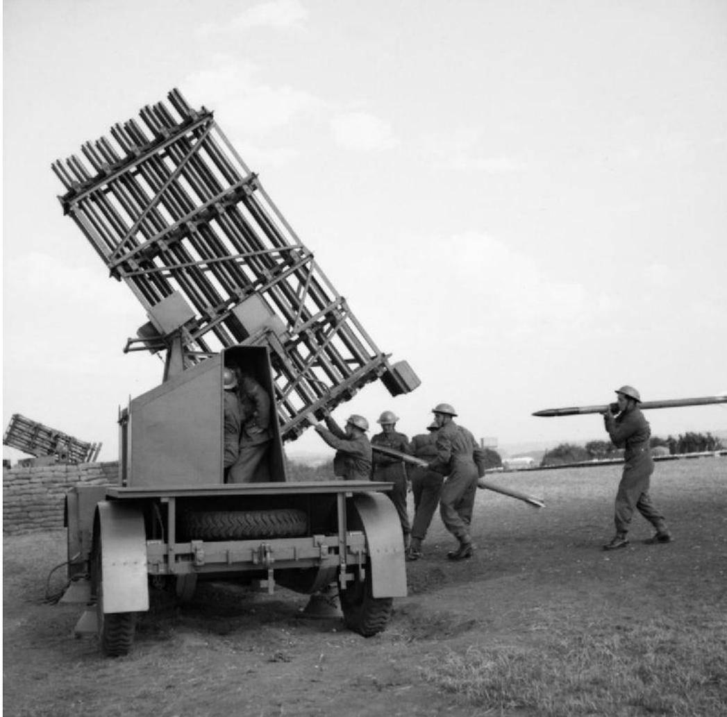
**2.3 Z-Battery Anti-Aircraft Rockets:** The Z-battery anti-aircraft rockets were deployed as early as 1941 to defend against German air attacks. The launcher fired 128 anti-aircraft rockets; The relatively simple to use system was used by British home guard troops. Launchers were also sent to North Africa where rocket launchers were mounted on towable trailers.
